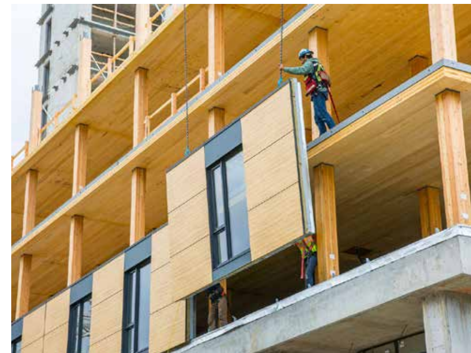
FIGURE 6-26: PRECEDENT IMAGE CLT CONSTRUCTION SOURCE: BROCK COMMONS, UBC
