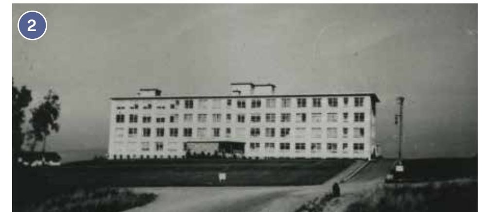
FIGURE 3-5: BURNABY GENERAL HOSPITAL, LOCATED AT 3880 INGLETON AVENUE, ONE BLOCK WEST OF GILMORE WAY, 1953 SOURCE: CITY OF BURNABY ARCHIVES
