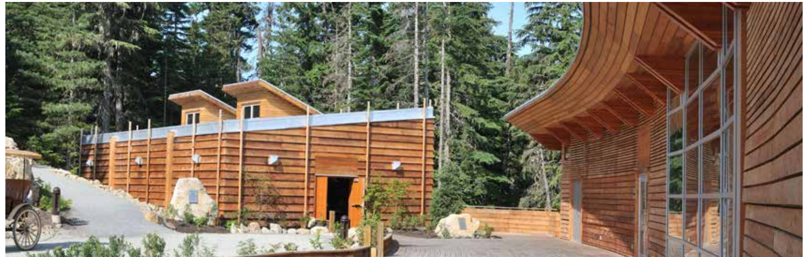
FIGURE 6-16: SQUAMISH LIL'WAT CULTURAL CENTRE MEZZANINE DECK 5,000 SQ. FT TOTAL (2,500 SQ. FT. IS COVERED) WITH CENTRAL FIRE PIT, WHISTLER
