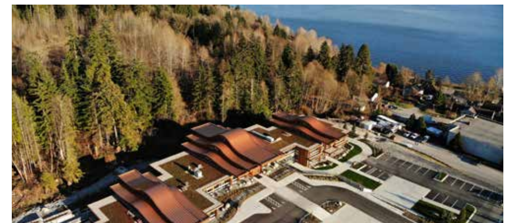
FIGURE 3-44: TSLEIL-WAUTUTH ADMINISTRATION BUILDING AND HEALTH HUB FEATURES RECYCLED MATERIALS AND WOOD SOURCE: SALISH SENTINEL
