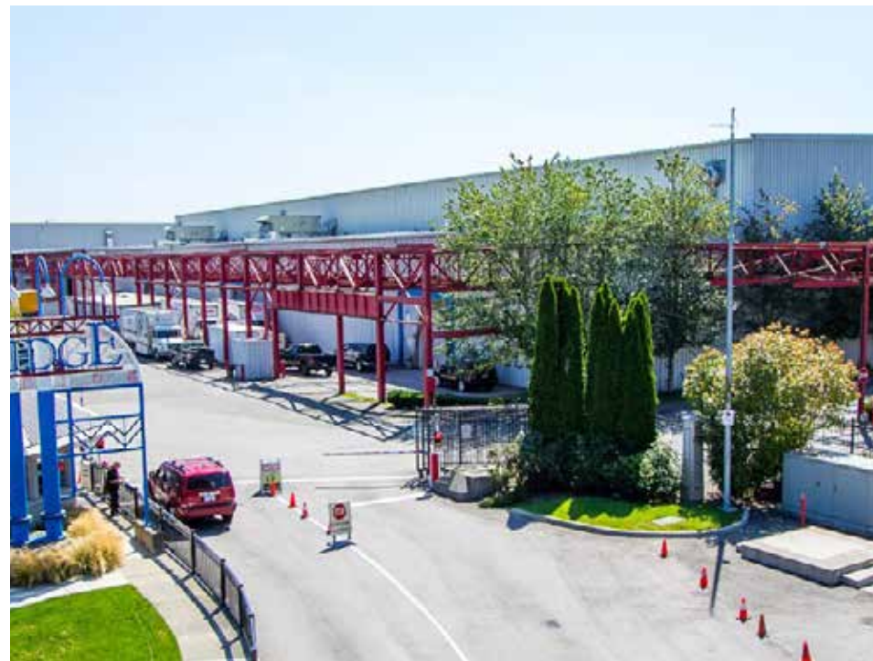
FIGURE 6-41: BURNABY STUDIO SOURCE: BRIDGE STUDIOS
