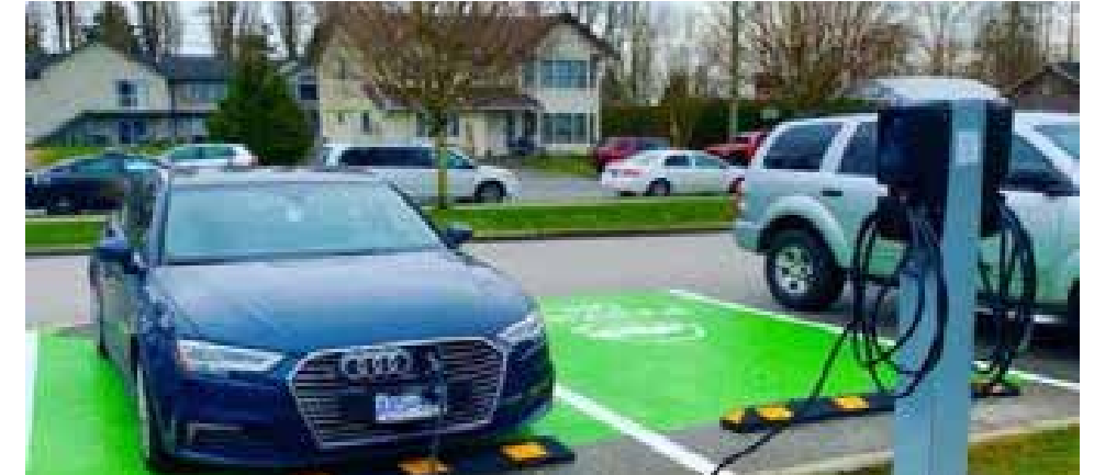
FIGURE 3-42: EV CHARGERS INSTALLED BY MUSQUEAM ADMINISTRATION SOURCE: MUSQUEAM
