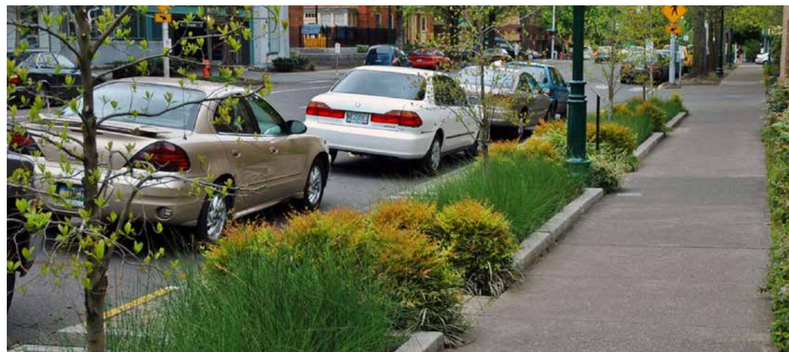
FIGURE 7-69: STREETSIDE STORMWATER GARDEN ON 12TH AVENUE IN PORTLAND, OR. SOURCE: PORTLAND, OR
